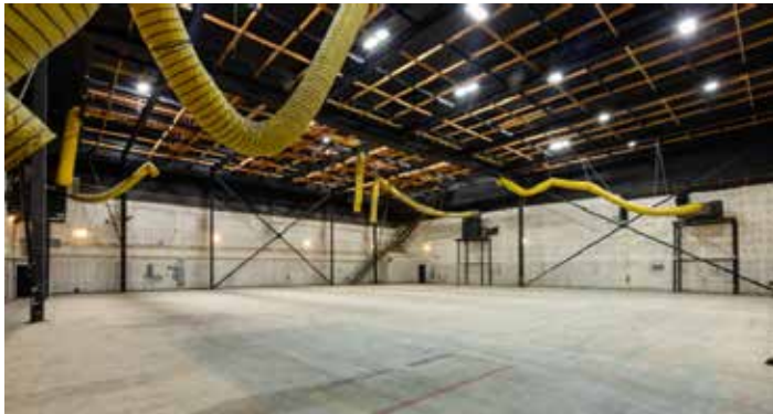
OVERALL RIGGING GRID
